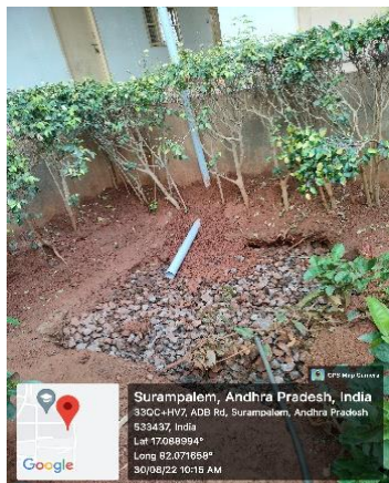
Construction of Recharge Pits
