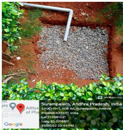
Construction of Recharge Pits
